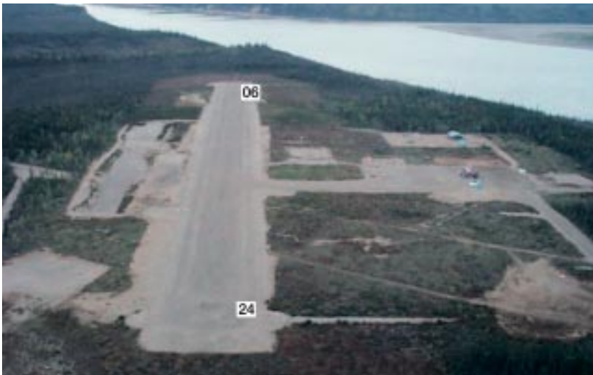
Photo 5-26 - Fort Good Hope looking southwest credit: Pryde Schropp McComb Inc
